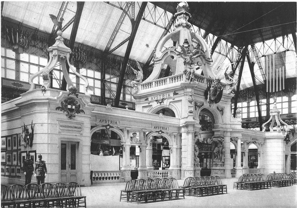
AUSTRIAN EXHIBIT.—MANUFACTURES BUILDING.
