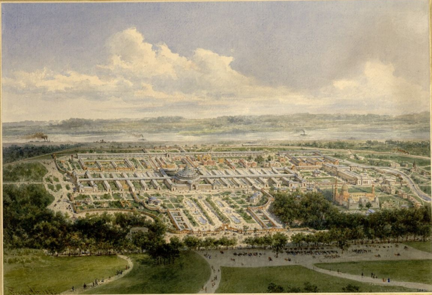
Franz Alt (AT), Exposition grounds at World Exhibition in Vienna, 1873 , Albertina, Vienna
