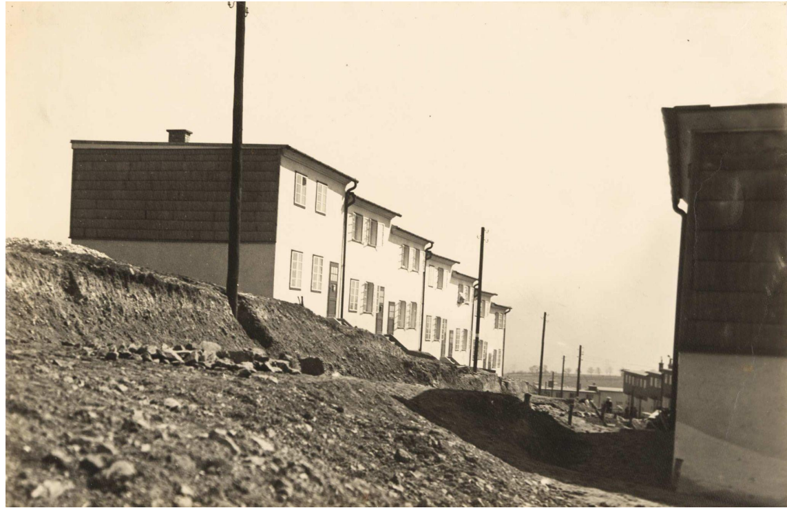
Estate "Heuberg" under construction, Vienna, circa 1926, Wien Museum
