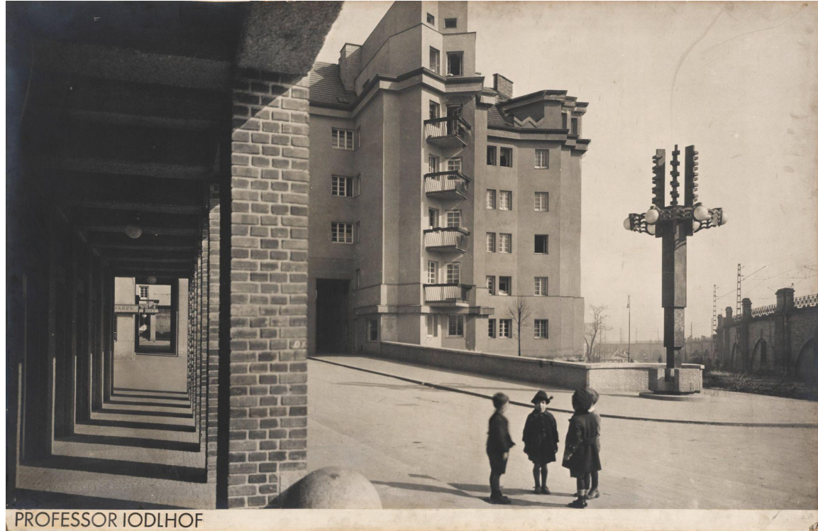
Municipality building “Professor-Jodl-Hof”, Vienna, photo by Martin Gerlach jun. (AT), around 1926, Wien Museum
