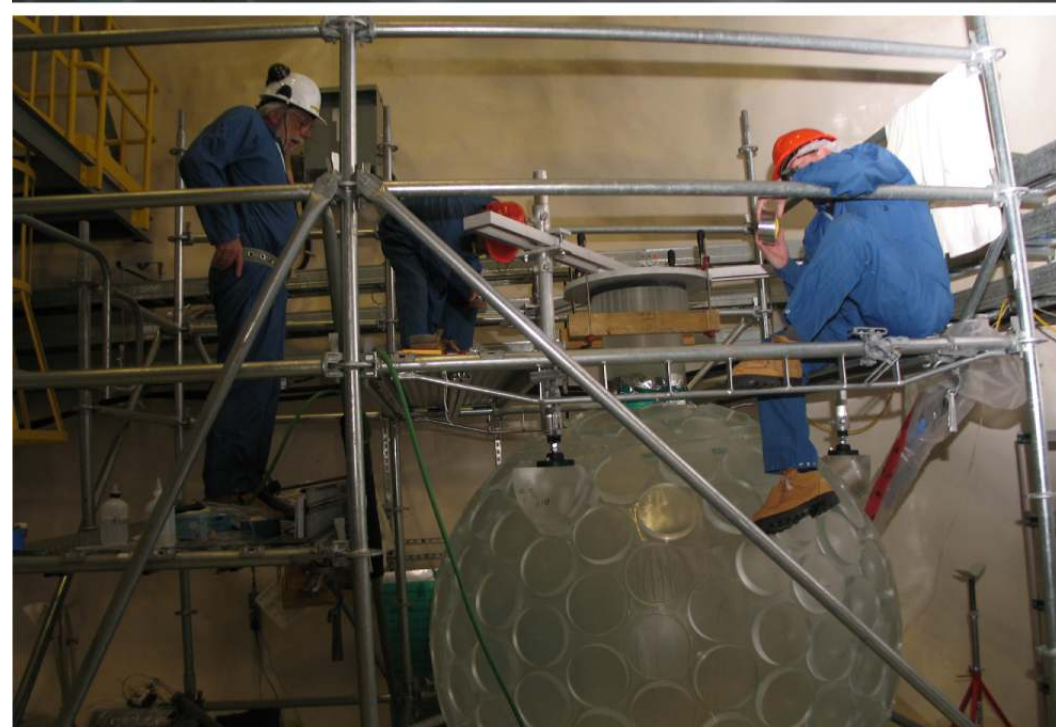
An RPT technician is preparing the AV for the collar bond.
