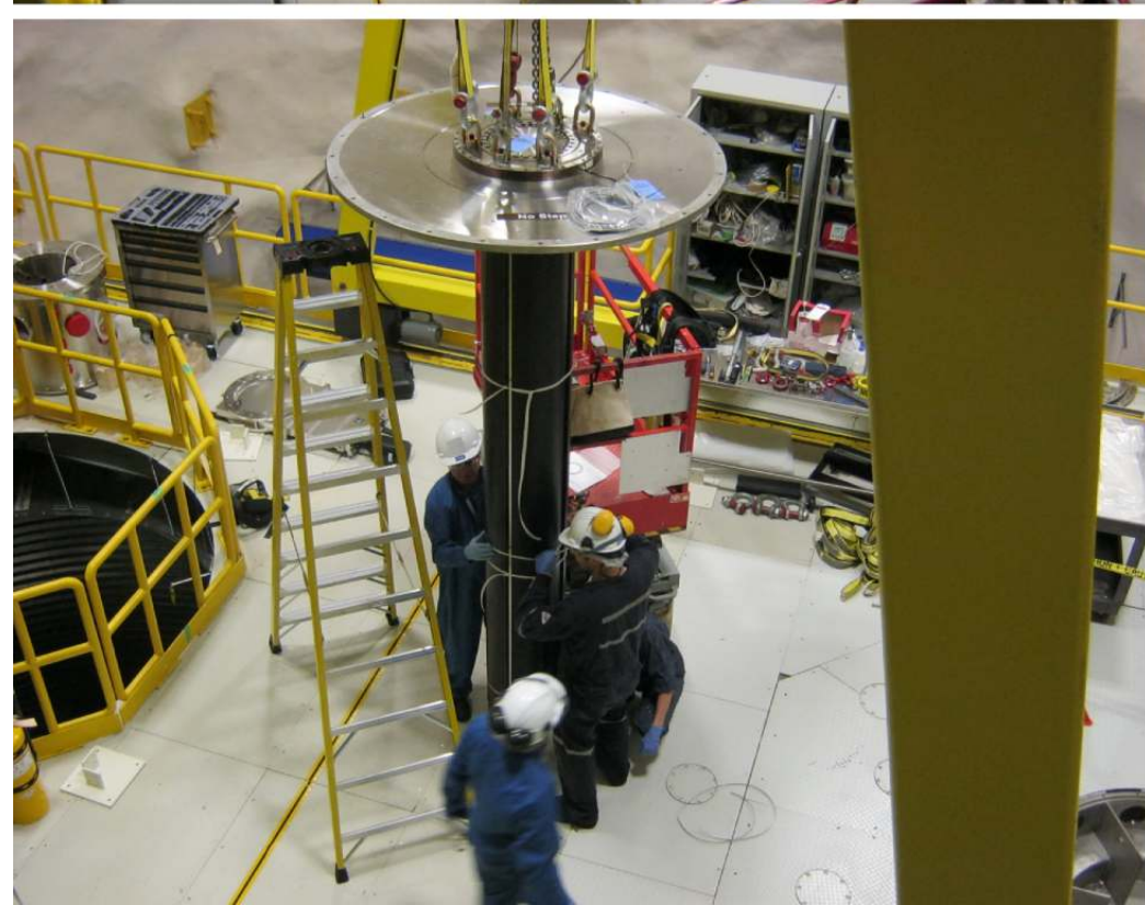
PMT and instrumentation cables strung through the neck.
