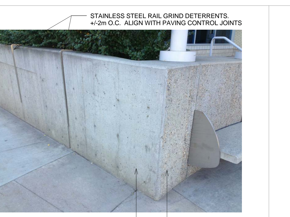
KEYNOTE A: FACE OF CONCAVE CURVE TO BE LIGHT SANDBLAST CONCRETE. ALL OTHER RETAINING WALL FACES TO BE SMOOTH CONCRETE. STAINLESS STEEL RAIL GRIND DETERRENENTS AT +/-2m O.C. (SIMILAR TO SOUTHEAST CORNER OF 87th AVENUE & 114th STREET INTERSECTION)
