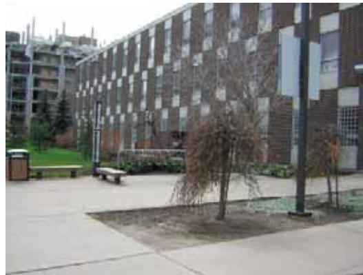
Figure 18 - Entry to Environmental Engineering
