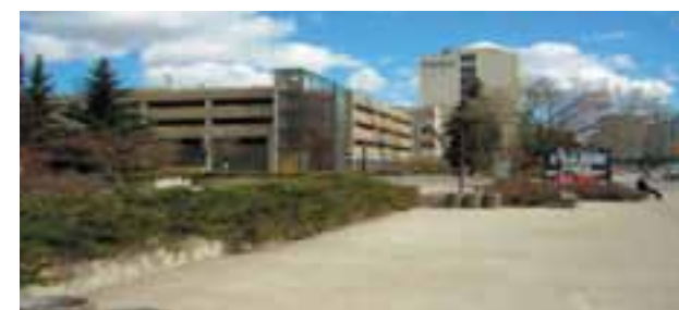
Figure 43 - Looking east toward the Education Car Park from Universiade Plaza
