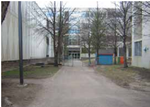
Figure 50 - Looking south toward the entry to the Education Courtyard East
