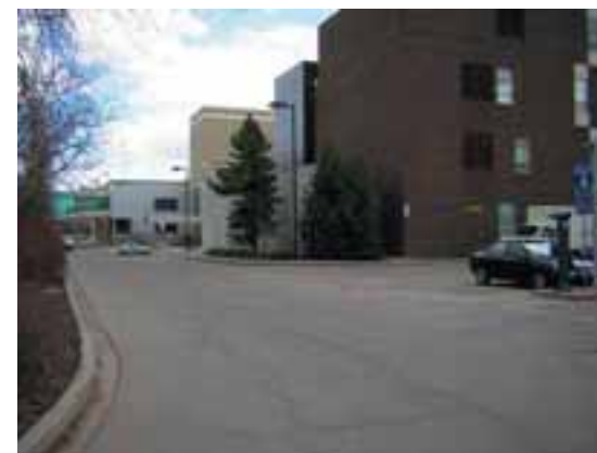
Figure 37 - North-west corner of the Environmental Engineering Building
