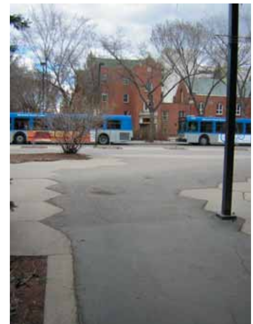
Figure 25 - Hard surfacing treatments at the north-east corner of University Hall
