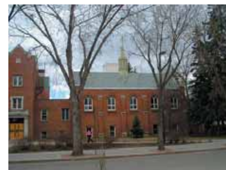
Figure 52 - West facade of St. Joseph's College
