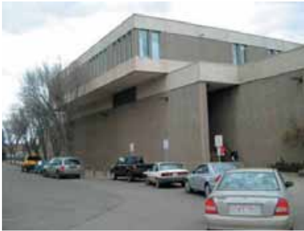
Figure 12 - Phys Ed East entrance from the north-east
