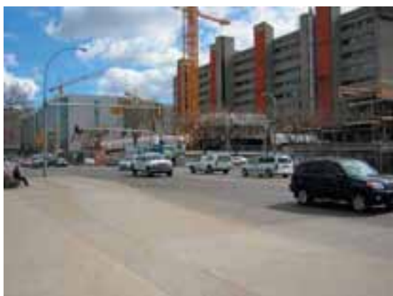
Figure 45 - Looking south-east at the intersection of 87 Avenue and 114 Street
