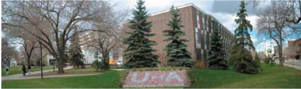
North-west corner of 87 Avenue and 112 Street - 'Before'
