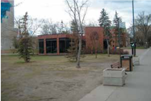
Figure 22 - LRT Access Building from the north-east
