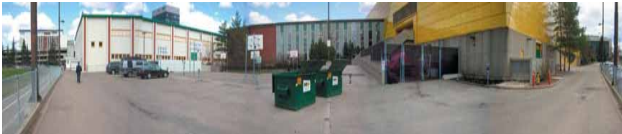
Figure 10 - Panorama of the Van Vliet Courtyard and service road
