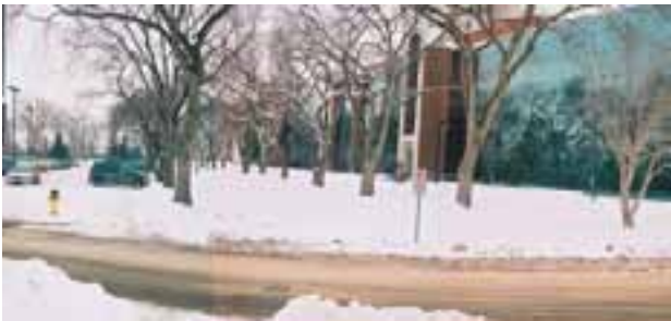
Figure 15 - Earth Sciences from the northwest at service road
