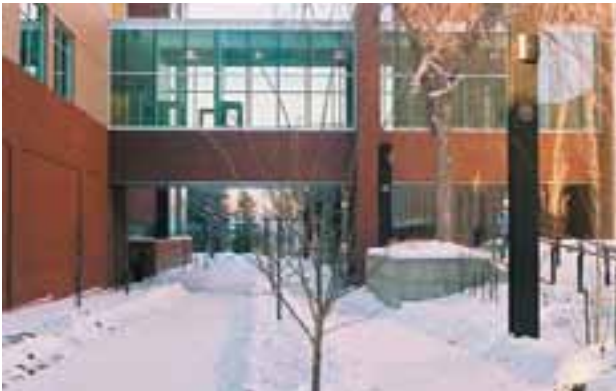
Figure 14 - Looking west at pedway between Chemical & Materials Engineering and ECERF/ETLC
