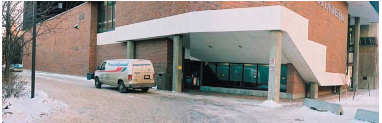
Figure 24 - North-west corner of Mechanical Engineering Building
