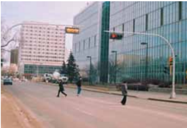
Figure 6 - North face of HMRC looking east along 87 Avenue
