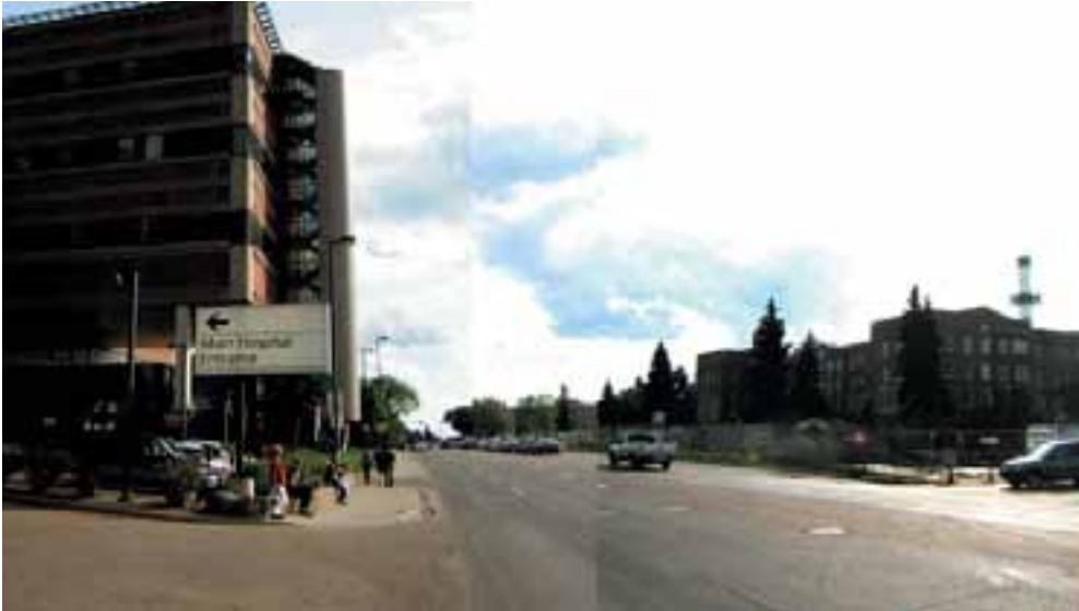
Figure 13 - WMC edge conditions north of 83 Avenue, looking south
