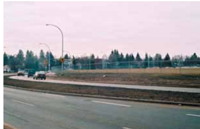
Figure 12 - Chainlink fence perimeter along Whyte Avenue
