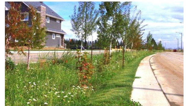
Storm water retention area integrated with roadway – in the neighbourhood of Magrath
