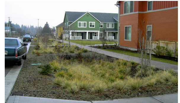
Storm water retention area integrated with sidewalk
