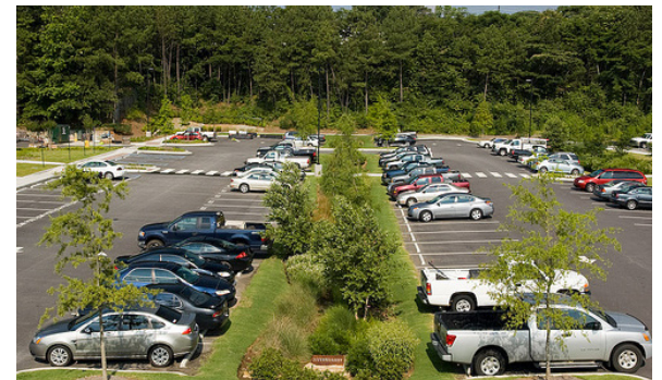
Storm water retention area integrated with surface parking
