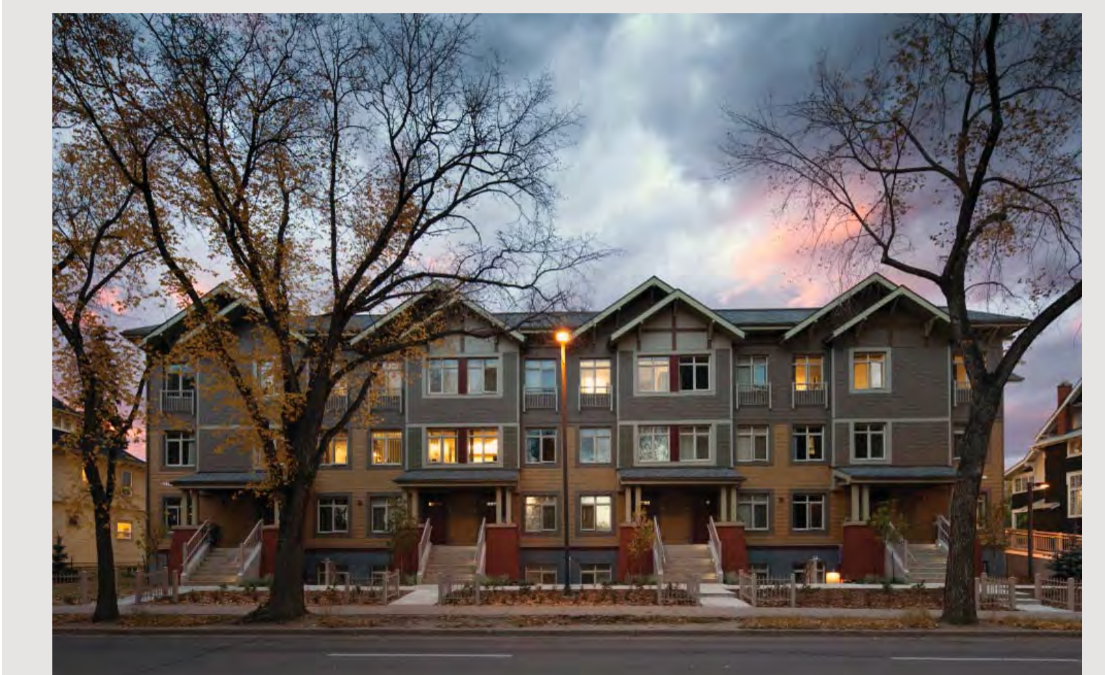
Student residences in a townhouse format (University of Alberta North Campus – Edmonton)
