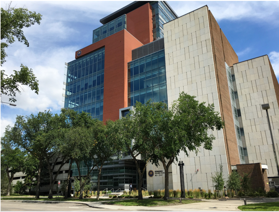
Donadeo Innovation Centre for Engineering (ICE), home of the NSERC Industrial Research Chair in Strategic Construction Modeling and Delivery. UNIVERSITY OF ALBERTA/ CASSANDRA OMMERLI
