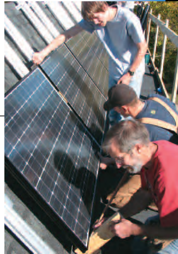
Solar electricity modules being installed.
