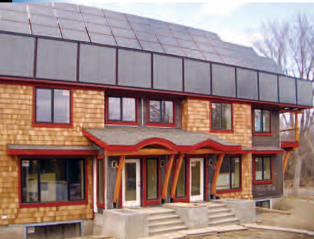
Riverdale NetZero House nearing completion.
