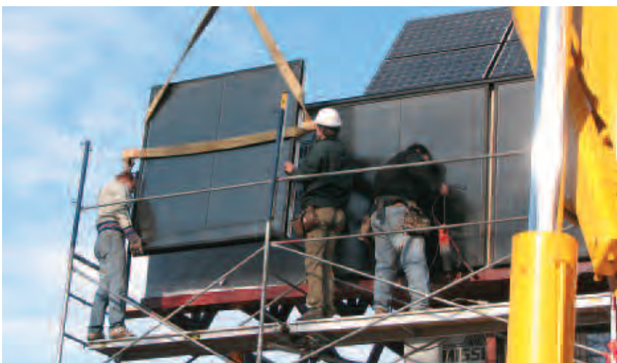
Solar heating collectors being installed.
