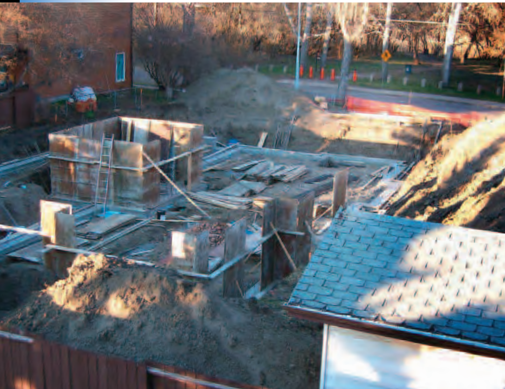
Basement forms showing solar heat storage tanks.
