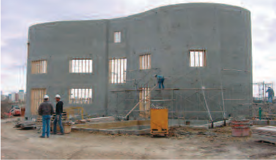
Unique structural concrete blockwork.
