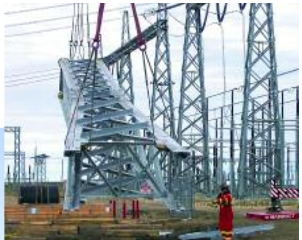
A powerline project by a Churchill company.
