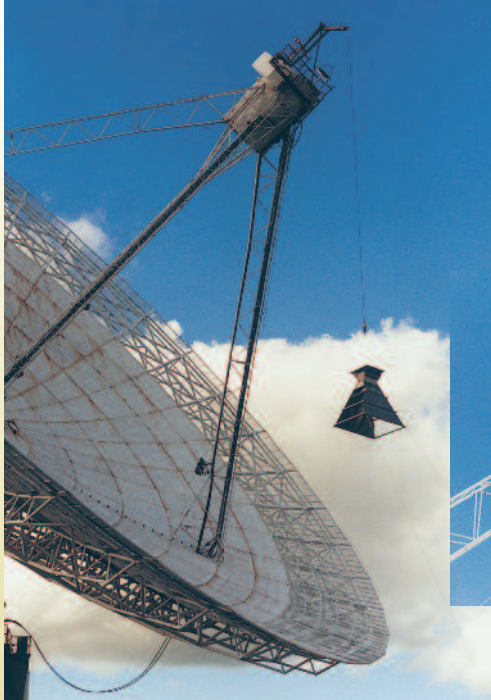
Left: The ridged feed horn is being winched up into the 46-metre diameter parabolic dish antenna at Algonquin Park in Ontario.
