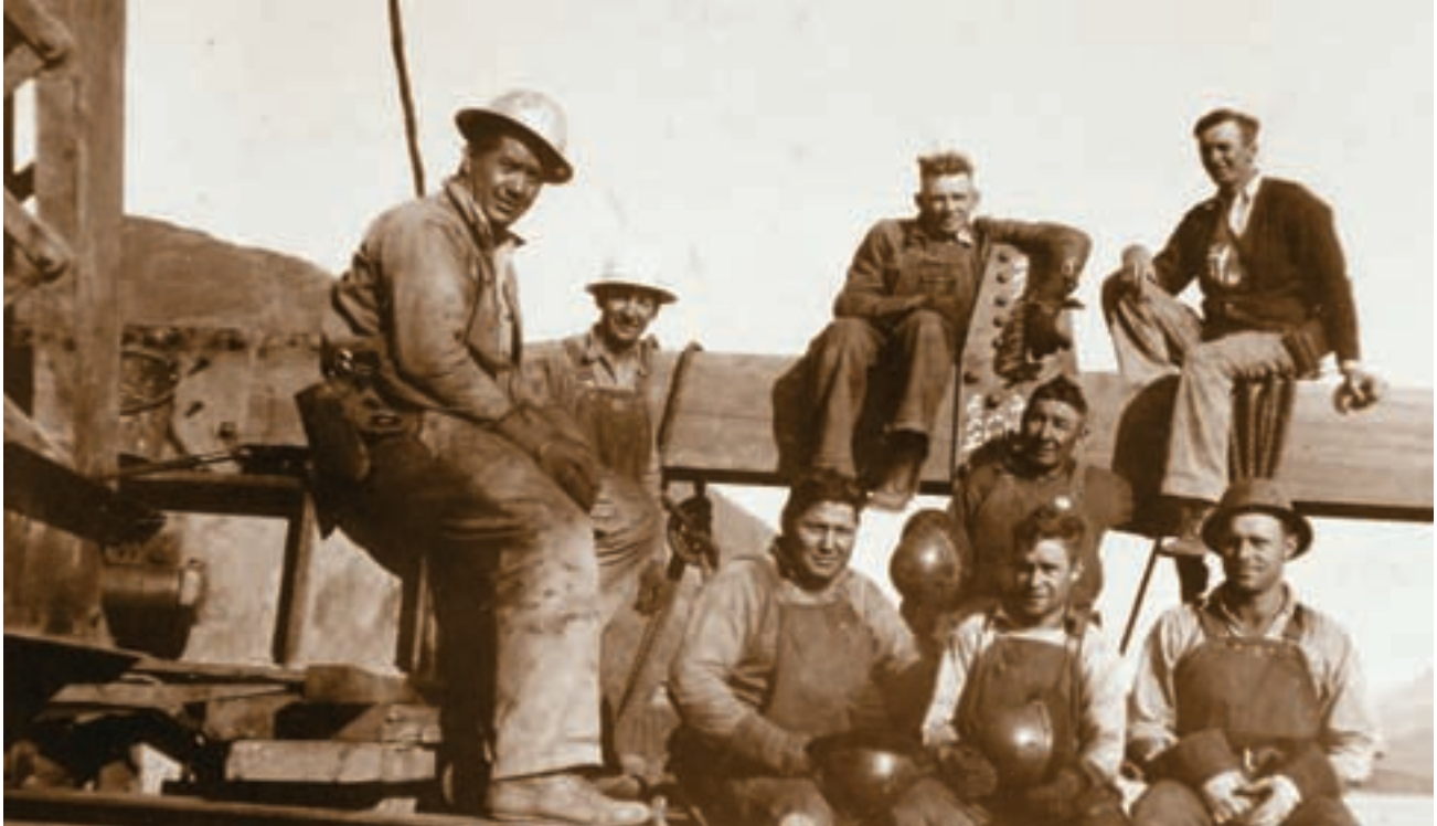
Liard Bridge, 1943. The rivet crew from New York.
