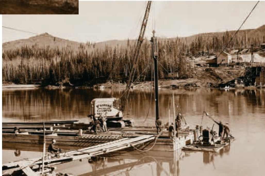
Alaska Highway, 1943. Laird River Bridge. Driving sheet piling at Pier 1.
