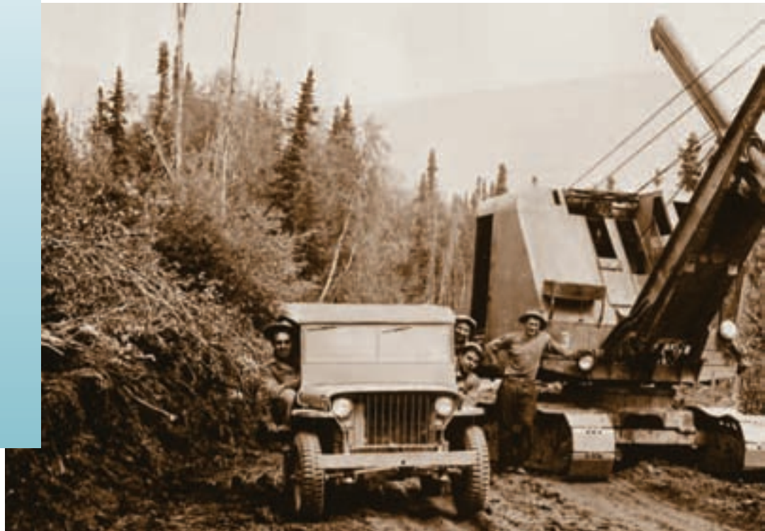
Alaska Highway Section D, with an army jeep and Osgood shovel.
