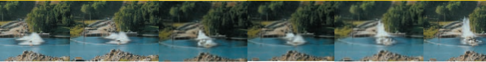
Sequential pictures of a marine pipeline blast.
