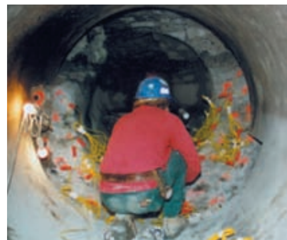
Enlarging a tunnel bore by blasting in Ottawa, Ontario.
