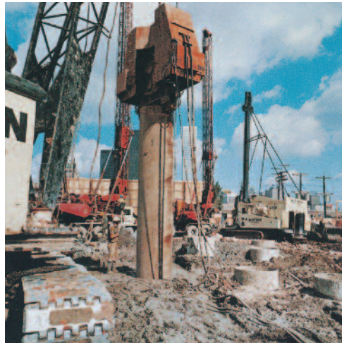
Left: Harbour Square Project in downtown Toronto, showing vibratory hammer setting steel sleeves, power augers drilling out overburden, and a churn drill forming rock sockets.
