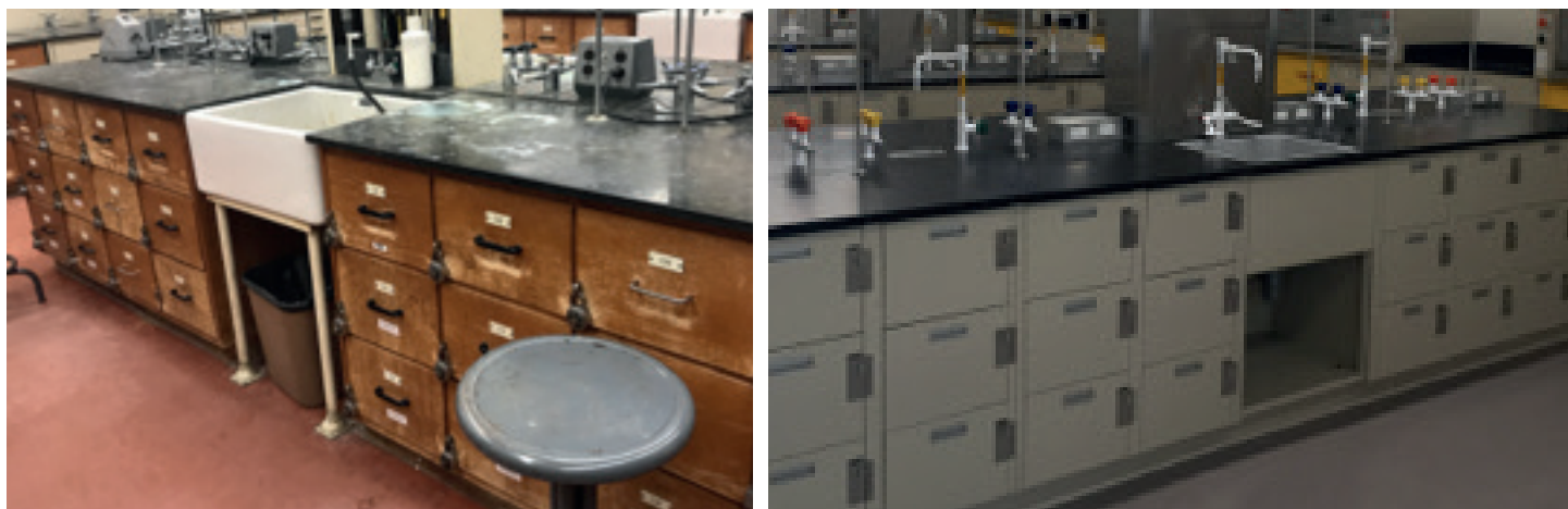
Undergraduate renovations before (left), and after (right)!
