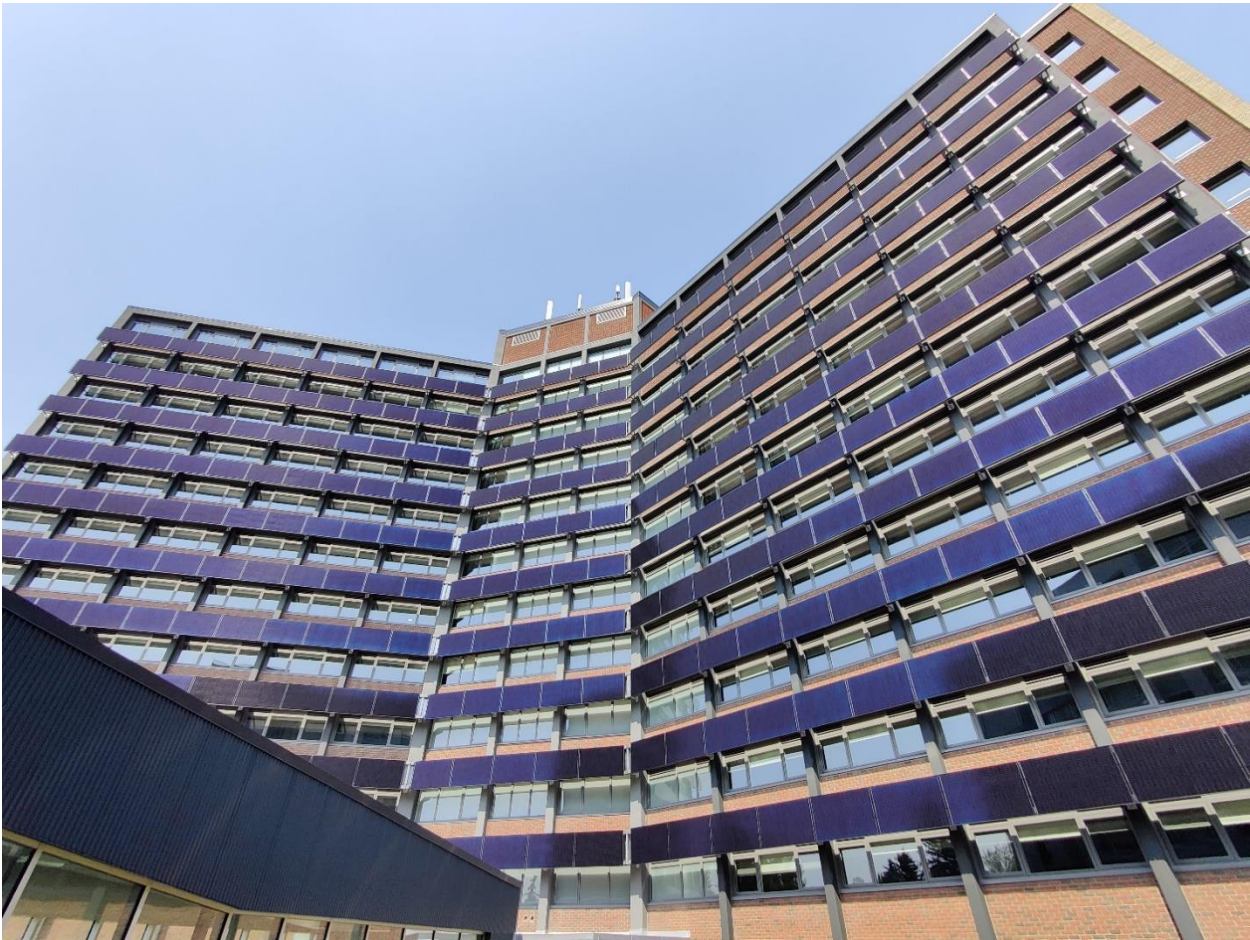
Figure 5. Lister Residence – Mackenzie Hall’s solar PV provides electricity and shade to reduce heat gain from the hall’s sunny south exposure.
