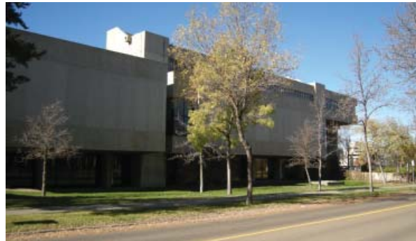
Figure 2.2 The Law Centre - North along 111 Street
