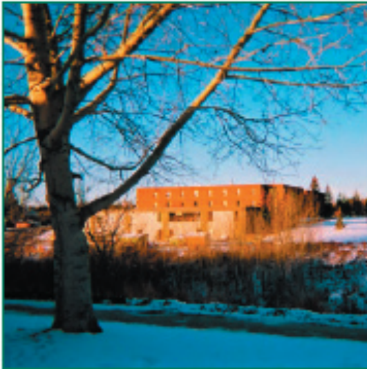
Auxiliary Building and Residence from east
