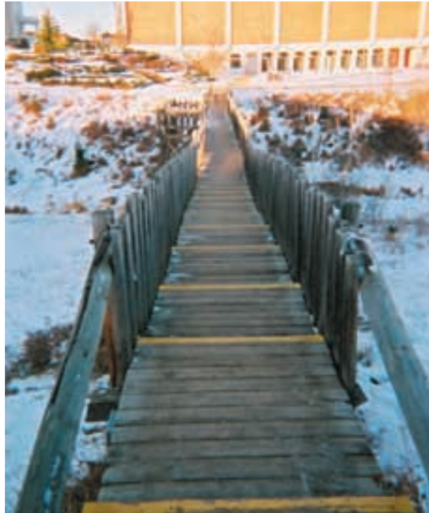
Bridge over creek ravine
