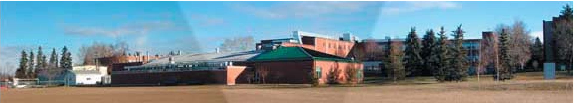
Figure 11 - View from the Recreation/ Open Space District looking northeast to Pavillon Central
