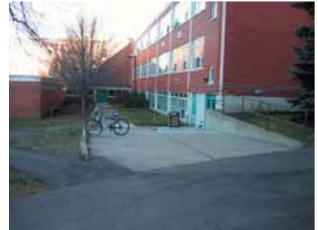
Figure 37 - Secondary Node at the south central access in Pavillon Central
