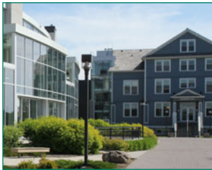
Renovation of Founders' Hall
