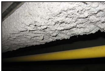
Spray-applied thermal insulation (fireproofing)
