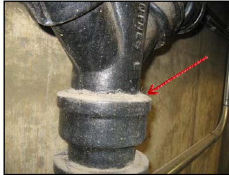
Joint packing on a cast iron pipe
