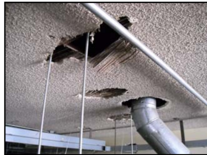
Ceiling texture coat
