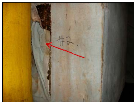
Parging cement on duct
