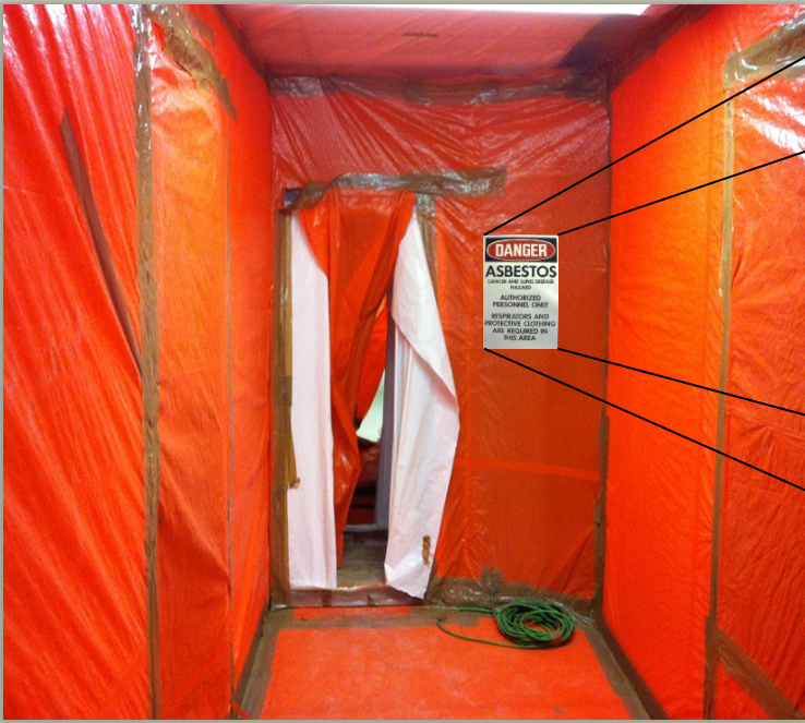
Typical entrance into an asbestos abatement containment (photo taken inside "Clean Room")
