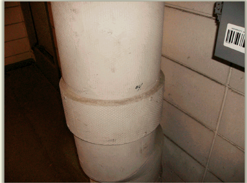
Cement (transite) fume hood exhaust duct – Chemistry Centre West
