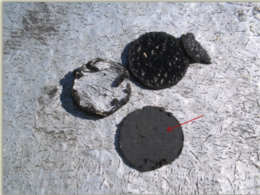
Roofing core sample (asbestos felt) – Triffo Hall (abated)
