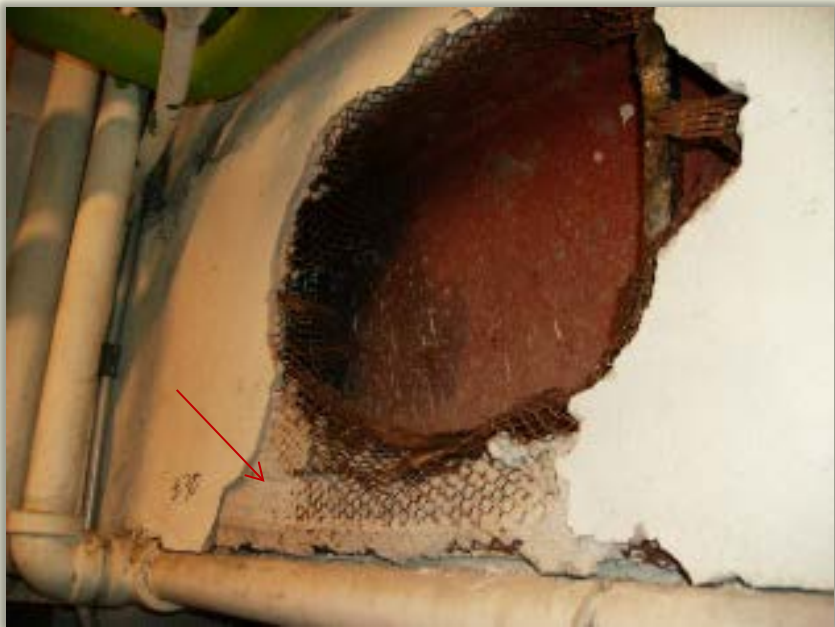
Plaster (rough coat) – Chemistry Centre West
