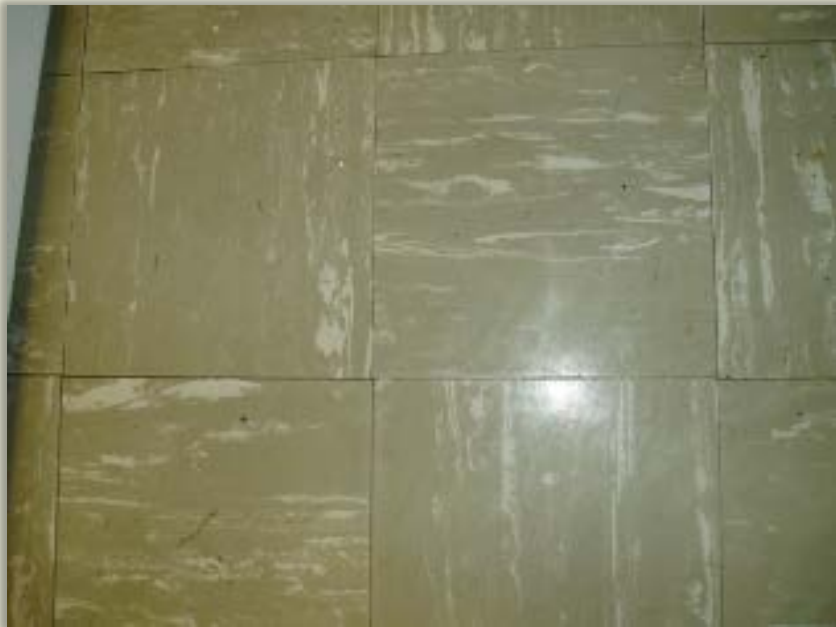
9"x9" vinyl floor tiles – Administration Building
