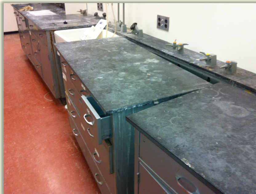
Countertop – Chemistry Centre - East
