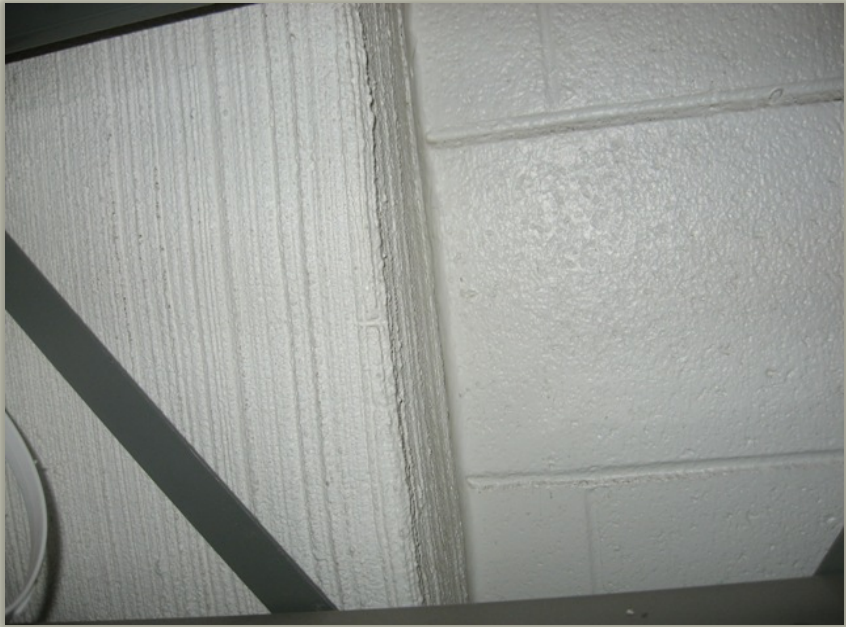
Trowelled Plaster – HUB Mall
