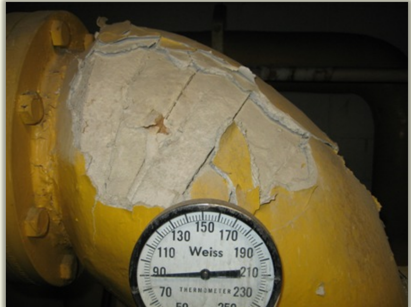
Pipe fitting insulation – Chemistry Centre East
