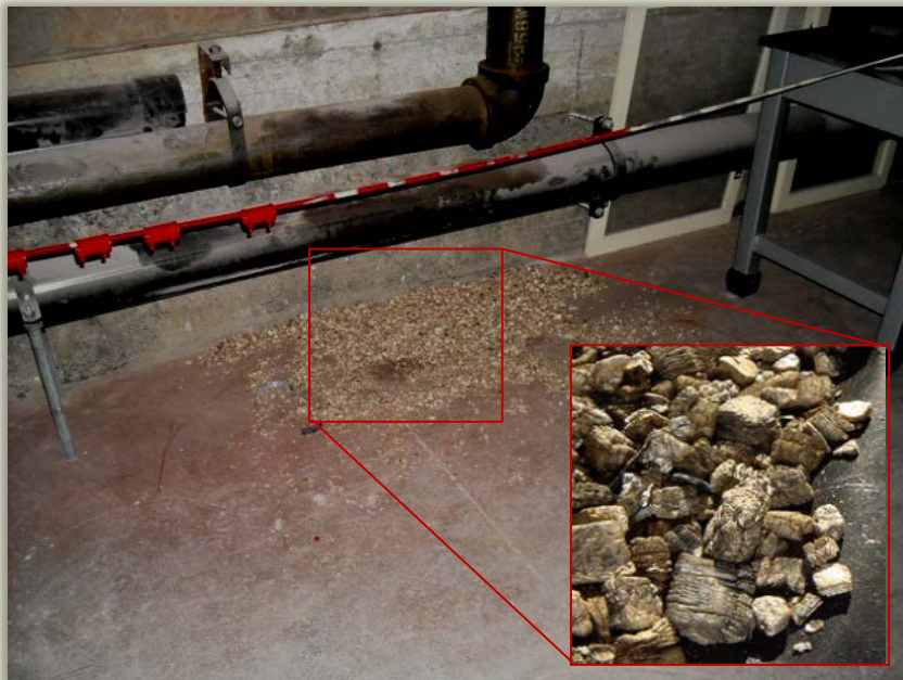
Loose brown vermiculite from block wall cavity – Chemistry Centre East
