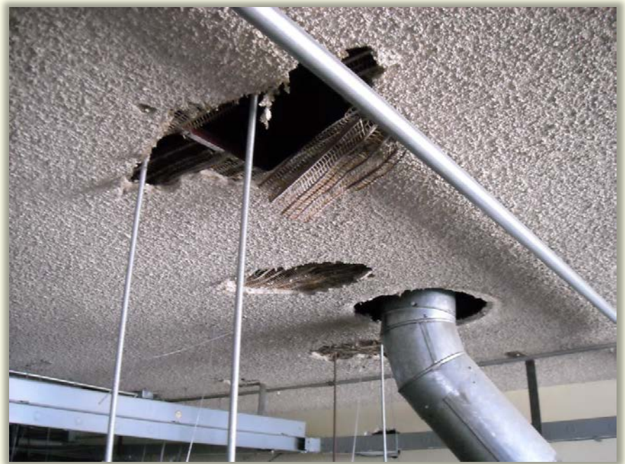
Spray-applied acoustical textured finish above T-bar ceiling tiles – Dentistry Pharmacy Centre
