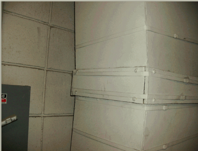
Cement (transite) fume hood exhaust duct – Chemistry Centre West
