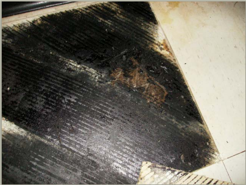
Floor Tile Mastic – General Services Building
