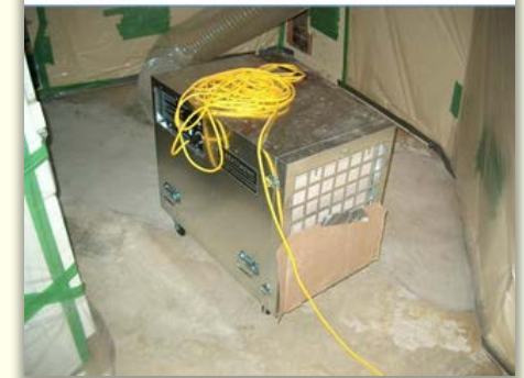
3-Stage Negative Air Unit (NAU)
