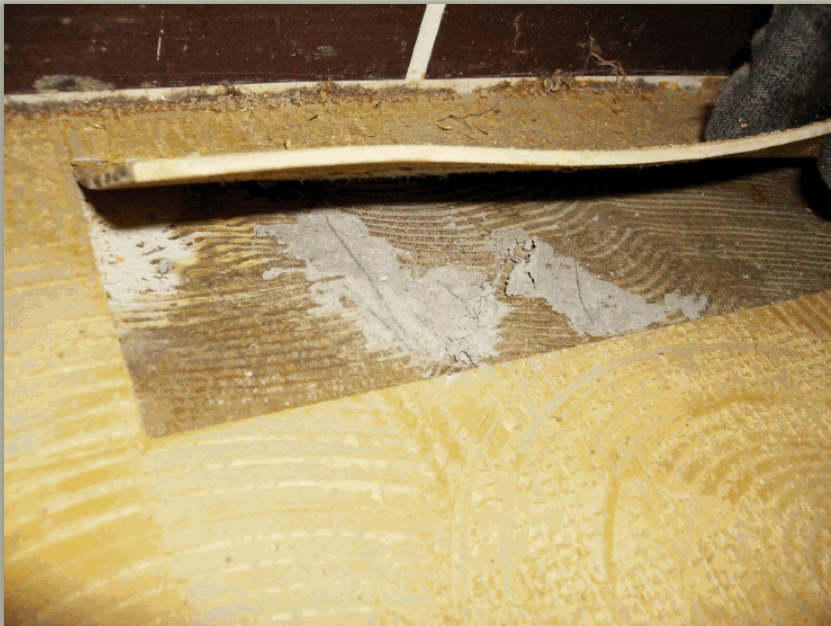
Fibrous floor levelling compound – Medical Sciences Building
