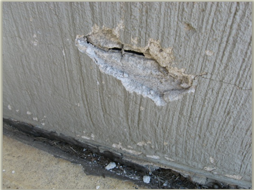
Trowelled Plaster – HUB Mall
