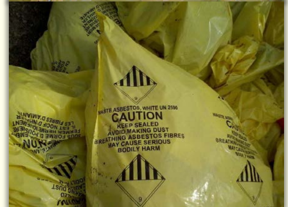
Asbestos waste bags used to store and transfer asbestos waste
