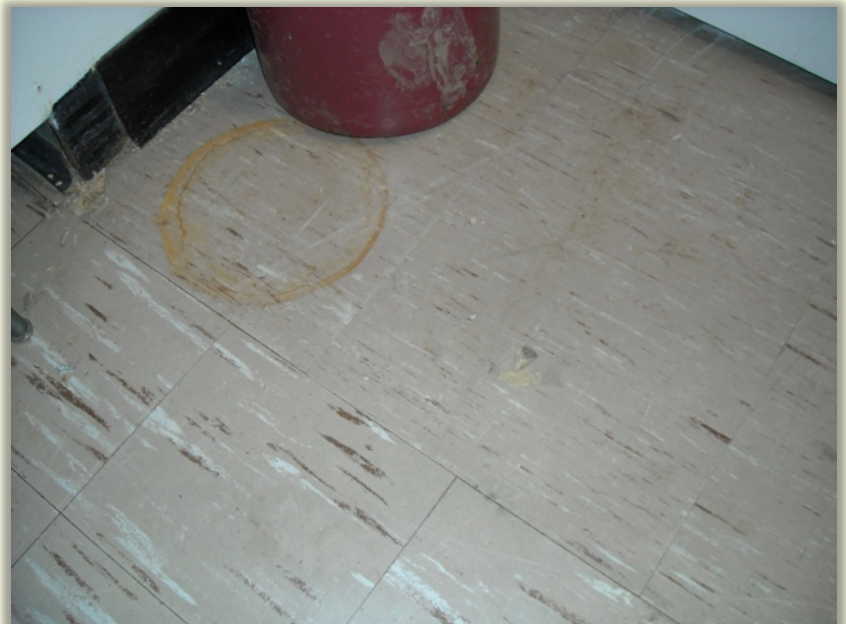
9"x9" and 12"x12" vinyl floor tiles – Chemistry Centre West
