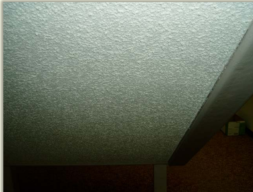
Decorative stipple coat – Mechanical Engineering Building
