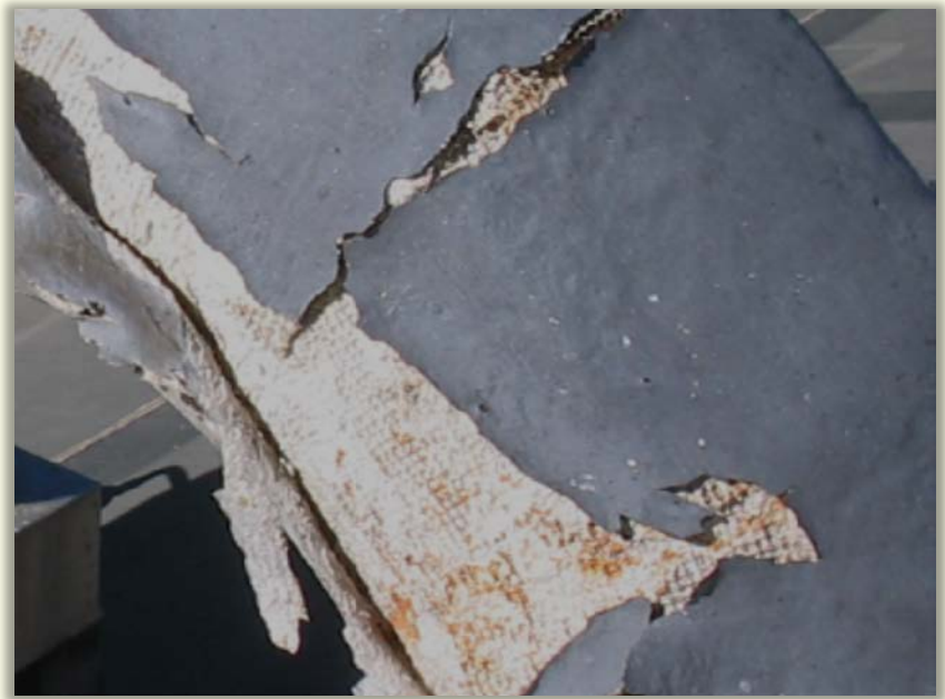
Felt on roof exhaust duct – Triffo Hall (abated)
