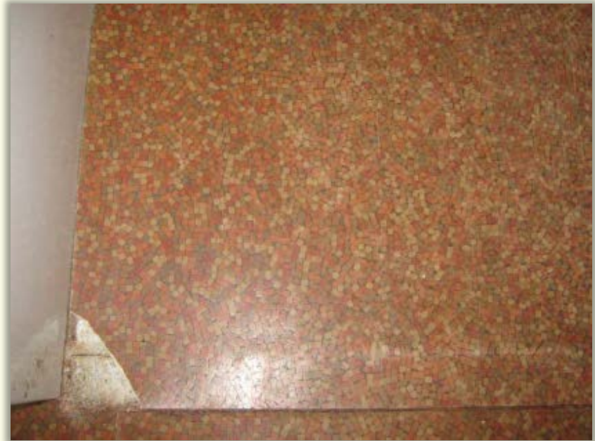
Sheet Vinyl Flooring – Chemistry Centre - East
