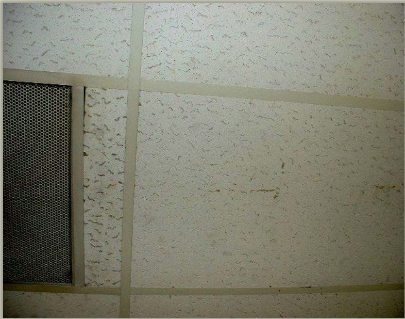
2'x4' T-bar ceiling tile – Medical Sciences Building
