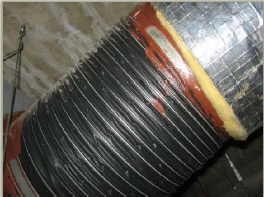
Mastic on ductwork – Chemistry Centre - East
