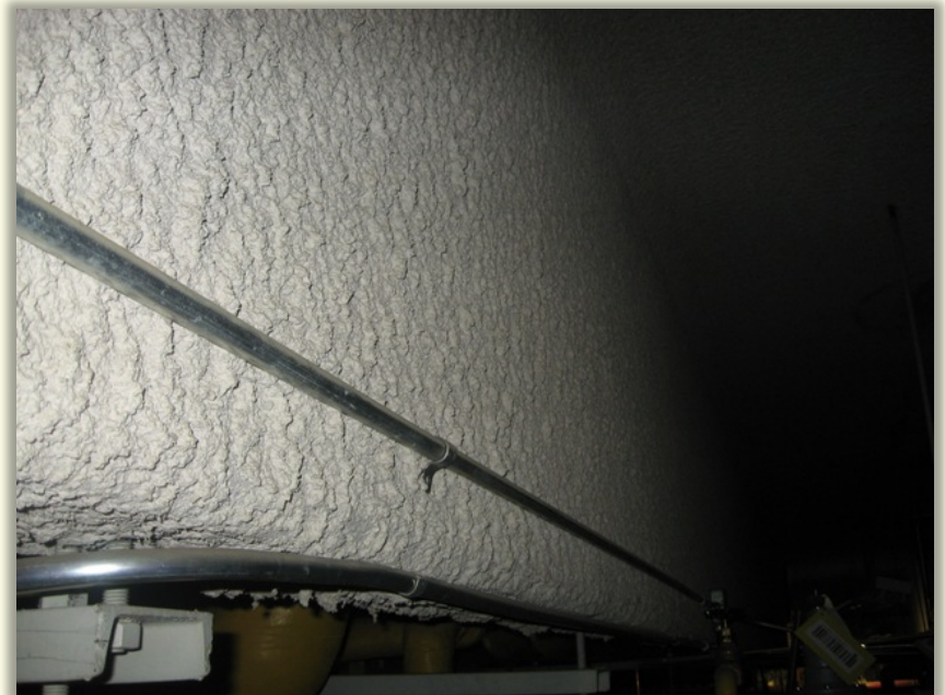
Spray-applied fireproofing – Chemistry Centre East
