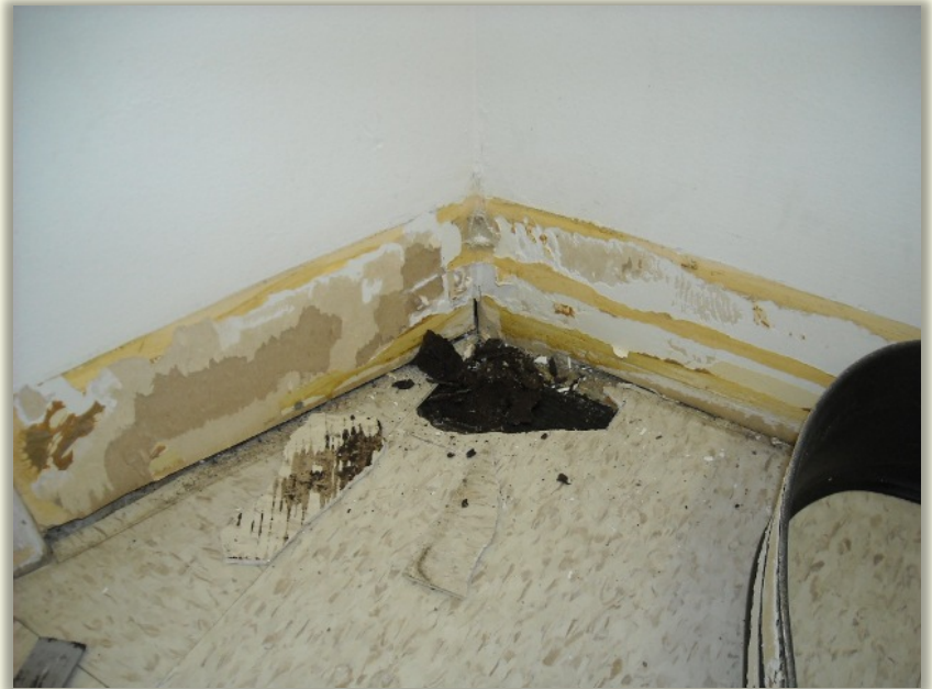
Cement-like floor levelling compound – Dentistry Pharmacy Centre
